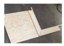
**18. FRAMING SHELF** Plan how you are going to layout your tile around the recessed shelf. Either dry lay the tile on the ground or draw out a diagram.
