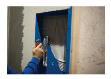
**8. SPREAD** Using the proper notched trowel apply thinset to the back of the shelf.
