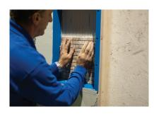
**9. SET** Lay the tile into the troweled thinset. Push firmly into the thinset. If needed use spacers to keep the tiles evenly spaced.
