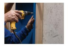
**4. SCREW** While keeping the shelf level screw the shelf into the studs and sleepers through the pre-drilled holes.
