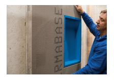
**5. BACKERBOARD** Measure and cut backerboard to fit around the shelf and cover your wall.
