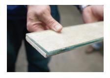
12. ANGLE CUT The recessed shelf is angled outwards on all sides so the water does not pool in the recess. The angle of the glass shelf mirrors the recess' angle. When cutting the sides of the recess use the glass shelf as a guide.
