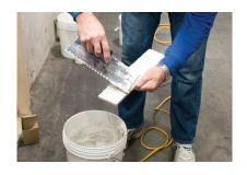
**14. SPREAD** When the legs are cut to size, use a notched trowel to apply thinset to the backside of the tile.
