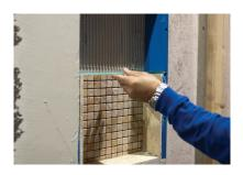
**16. SHELF** When all sides are installed below the glass shelf place the glass shelf onto the set tile and push it tight to the back of the recessed shelf.
