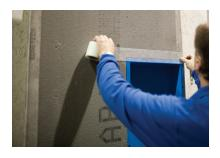
**6. FIBER TAPE** Use fiber tape on all sides of the shelf and on all of the cement board joints.
