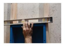
**3. LEVEL** Place in the recessed shelf in between the studs and the sleepers. Again use a level.
