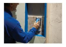
**10. FLOAT** Use a float to be sure that each of the tiles are evenly and firmly pushed into the thinset.
