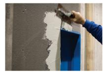
**7. SKIM** Using the flat end of the notched trowel, skim over the fiber tape. The thinset should be smooth and just thick enough to cover the tape.
