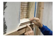
**20. PROFILES** The Tile Shop offers a variety of profiles to finish the edges of the recessed shelf. Use 45 degree angle cuts to form the corner joints. Always try to layout the frame using as long of profiles as possible
