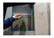
**11. MEASURE** Use a tape measure to determine the desired height of the glass shelf.
