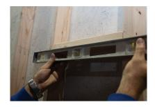
2. SLEEPERS Using 2x4's as sleepers, measure, cut and screw between the studs. Be sure to check that they are level
