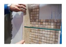
**17. TOP EDGES** Using the same techniques as steps 13-15 measure, cut and install the remaining tile sides and top of the recess.
