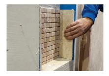
**15.SET** Press the tile firmly onto the recessed side.
