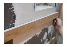
**19. GUIDE** Temporarily nail a piece of wood batten to the wall to prevent trim pieces from sliding.
